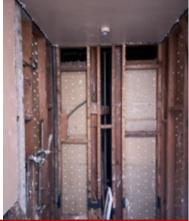
Inside one of the gutted spaces: corroded pipes, leaks, etc.
